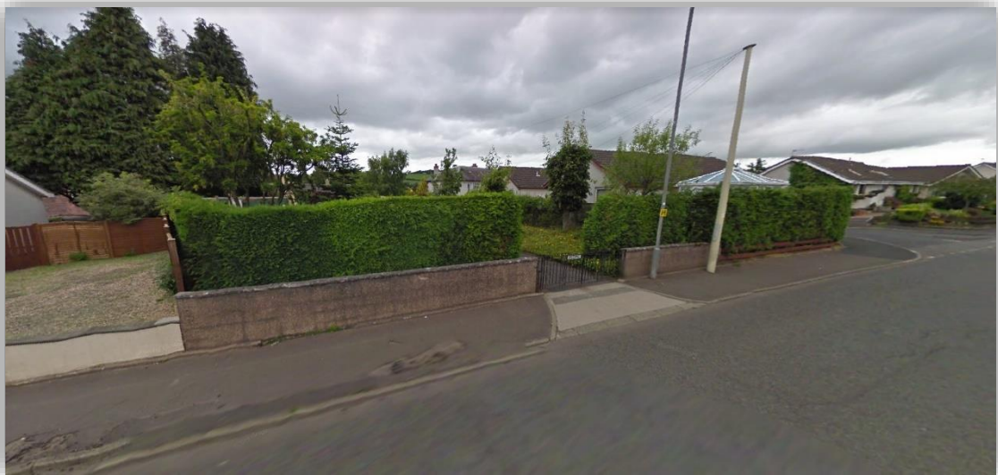
Figure 3: A streetview image of the site
